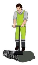
Shape and compact the surface carefully by tamping. The hardening can be expedited by adding water on the patched area at a ratio of 2 litres per 20 kg of asphalt repair compound. If there are a lot of spots that need patching or the areas are large in size, it is recommended to use a mechanical compactor. Individual small patches can be tamped with a spade, wide rubber mallet or simple hand ram. Driving over the spot a few times with a car also helps to compact the patch.
