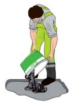
Pour compound from the container into the pothole until the surface is a few centimetres higher than the edges of the hole, depending on the situation. Do not overlap the compound with the asphalt.
